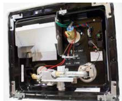
Water heater controls accessed from an exterior panel
