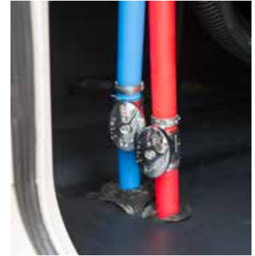
Typical low-point drain valves
