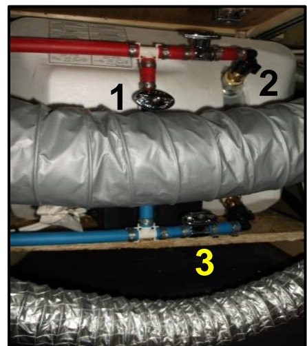
Figure 5 Water Heater Bypass Valves Location
