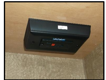
Figure 29 GFCI Plug in Bathroom above Toilet
