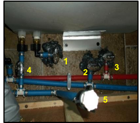
Figure 6 Low Point Drains (under passenger side bed)
