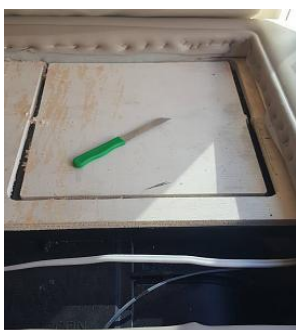
Figure 50 Access Panel Cut
