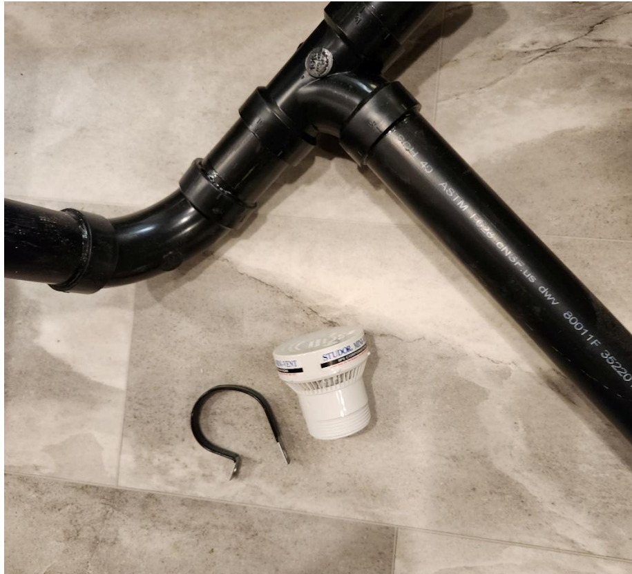
Figure 10 Save the clamp and air admittance valve
