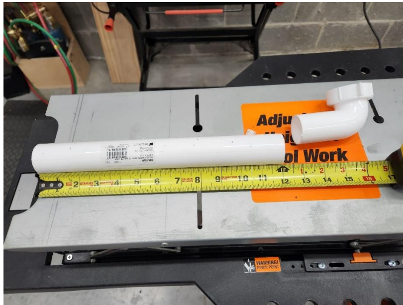
Figure 11 Cut waste arm 12 inches from the end
