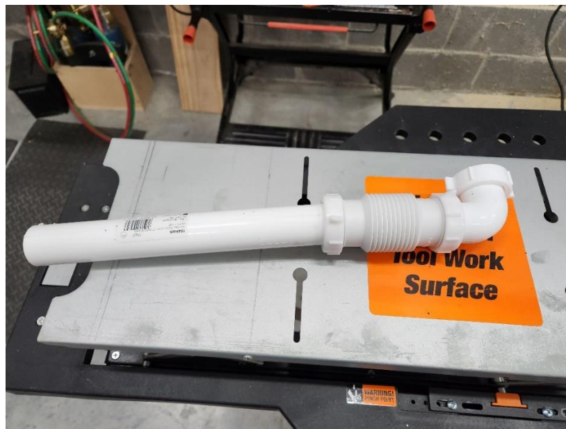
Figure 12 Use the flexible coupling to reconnect
