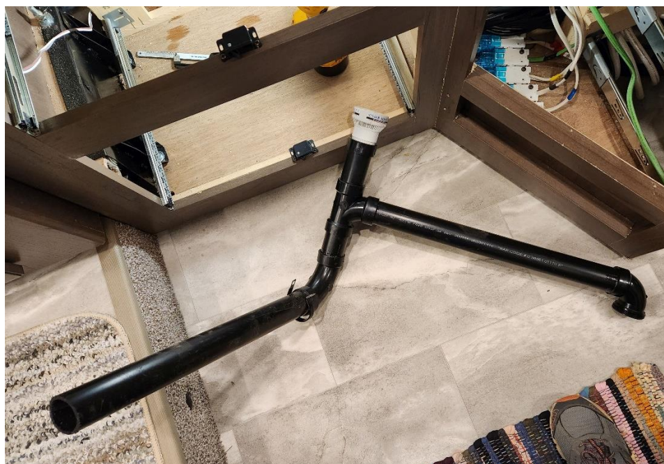
Figure 9 Remove P-trap and old section of drain pipe
