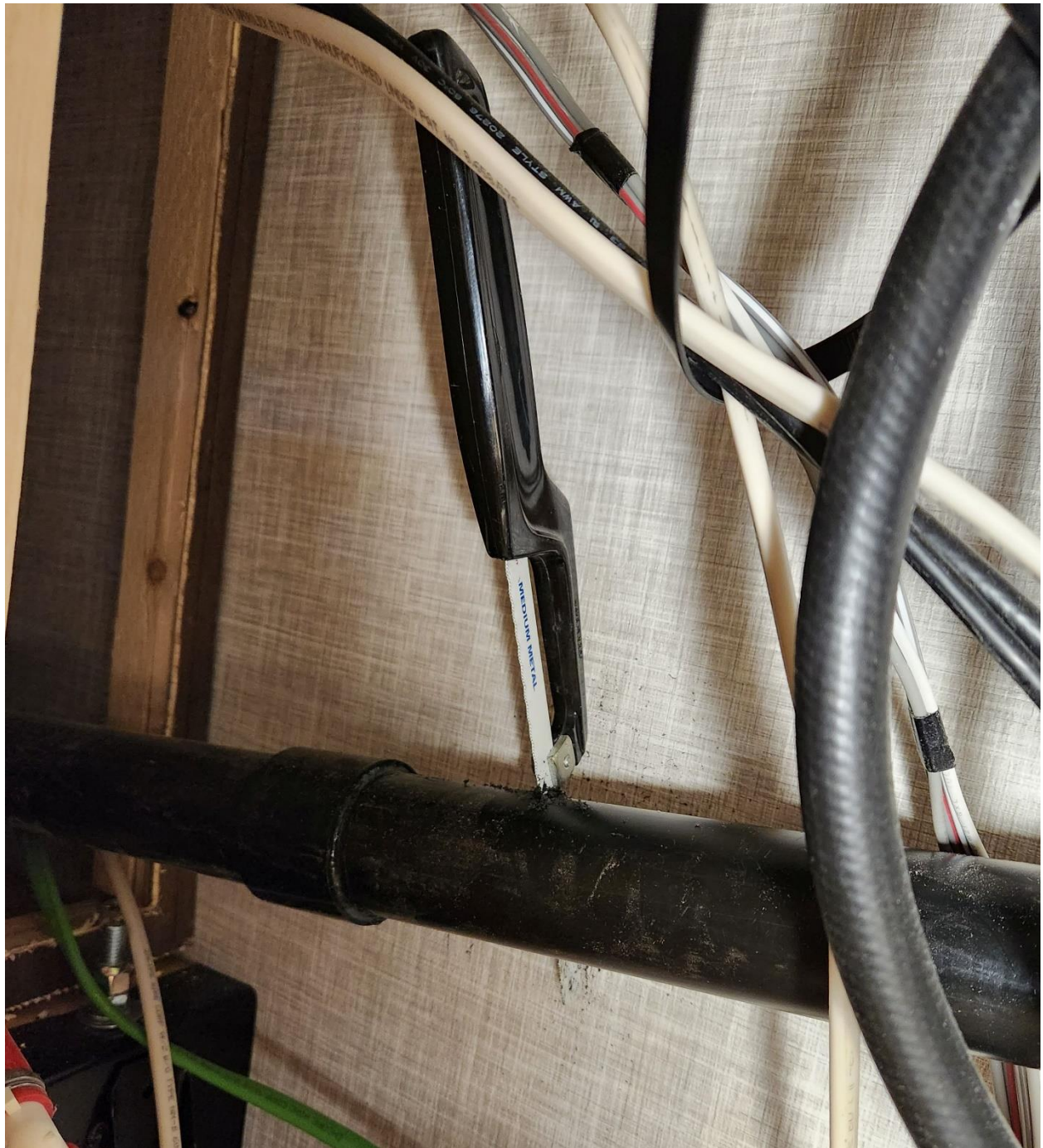
Figure 7 Saw pipe about 3 inches in front of existing joint
